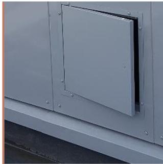
Weatherproof access hatch for ongoing maintenance
