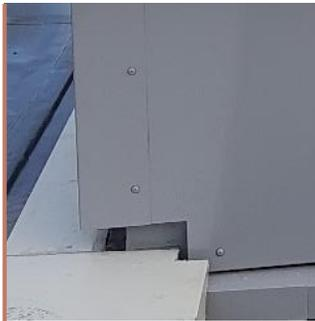
Bespoke Weathering detail for interface with parapet wall
