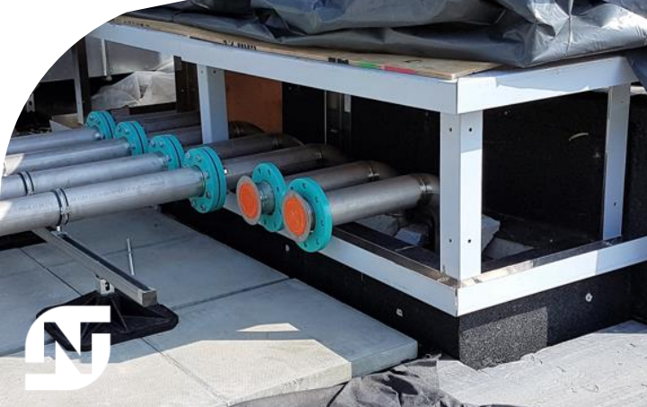
Modular frame with services installed onto the roof area
