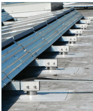
Retrofit to existing roofing
